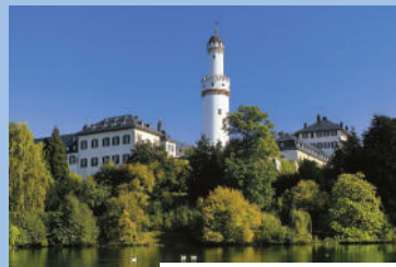
The baroque Landgraves' Castle was built between 1678 and 1686. Only the White Tower in the castle yard is left to witness the previous medieval building.
